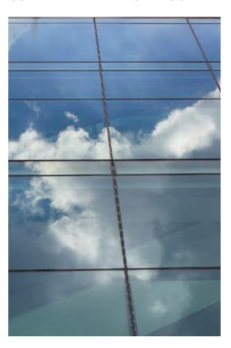
Post-bar facade glazing is the most common variant of stained glass glazing facades. It is a vertical and horizontal aluminum profiles. The space between is filled with single glass in a cold facade or a multi-layered glass unit in a warm one.
